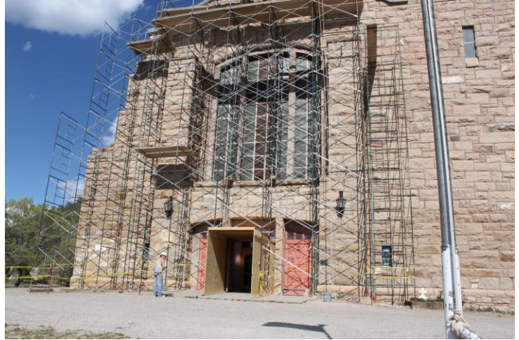
Gilbert checking out the scaffold
