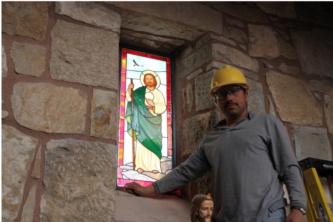
Martín Pizarro finishing the installation of the St. Jude window.
