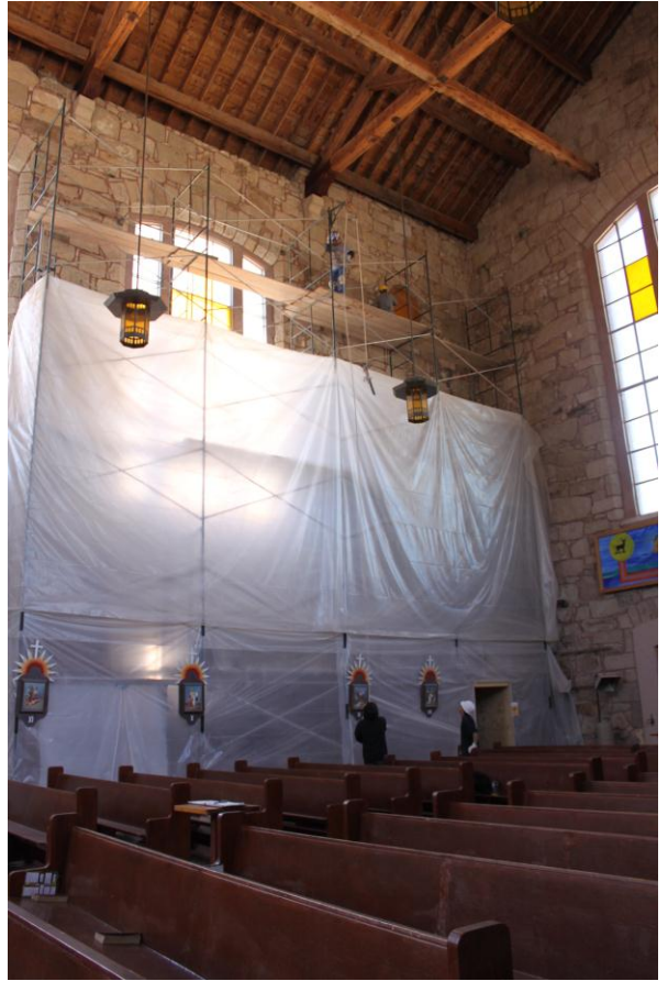
The crew removing the interior scaffolding
