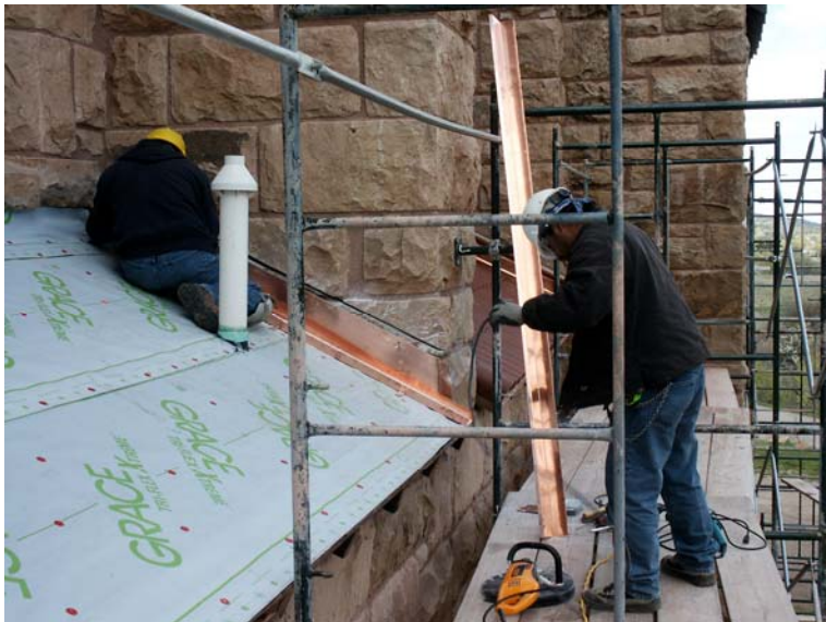
Martin Pizarro and Sam Sosa installing Copper flashing.
