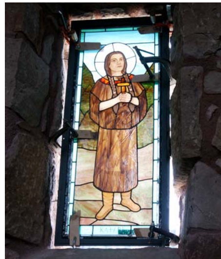
The Kateri stained glass window being installed.
