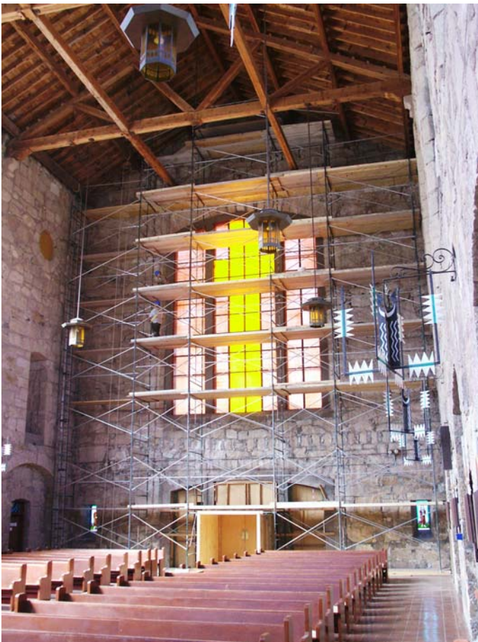
Scaffolding on west wall under construction
