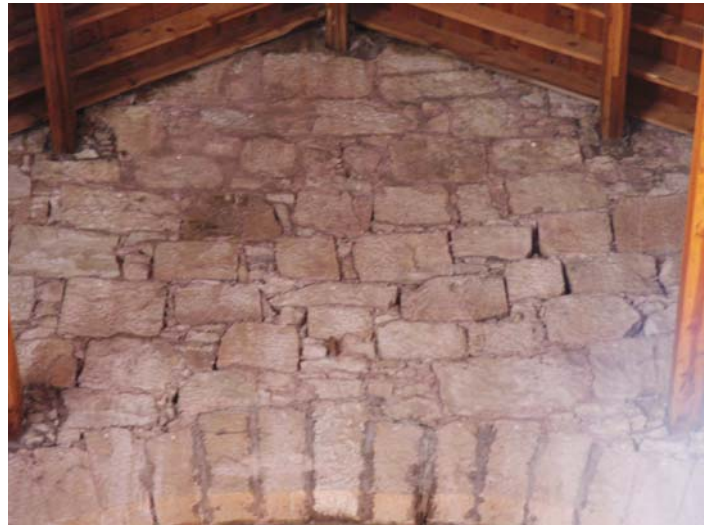
Top section of the West interior wall "before"
