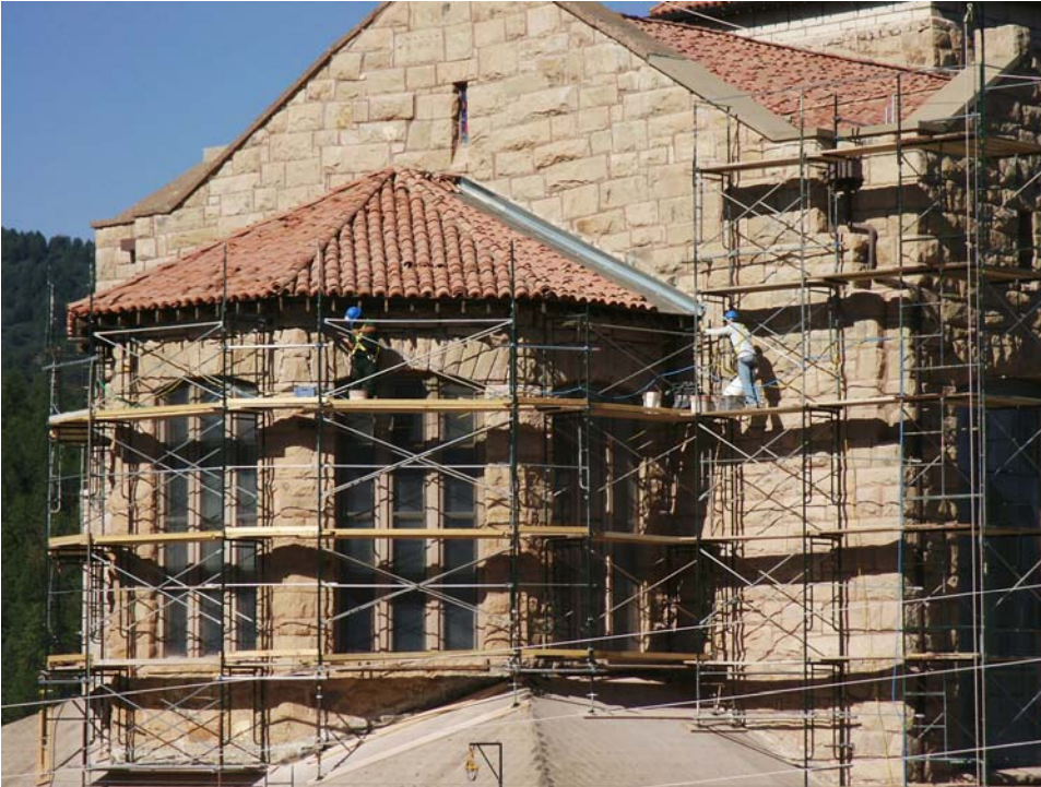
This summer we restored the apse exterior
