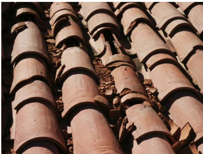
Roof tiles before removal from apse
